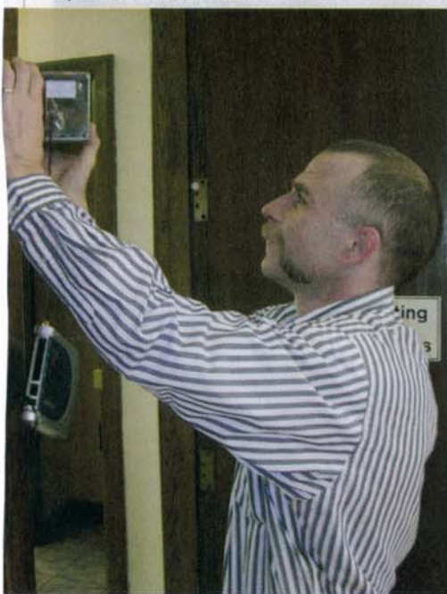
PHOTO COURTESY OF ARMIDA TECHNOLOGIES
