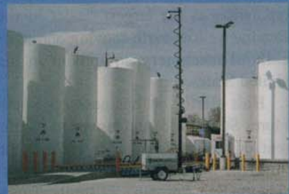
PHOTO COURTESY OF VICON INDUSTRIES INC.
